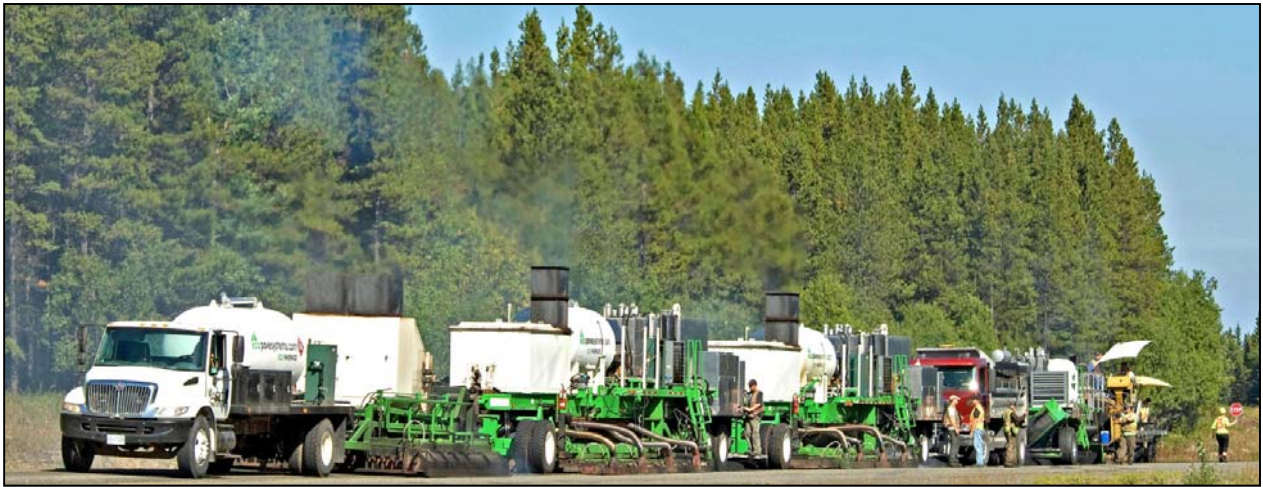
Figure 10. ARC Train Work In Progress on BC Highway Project
