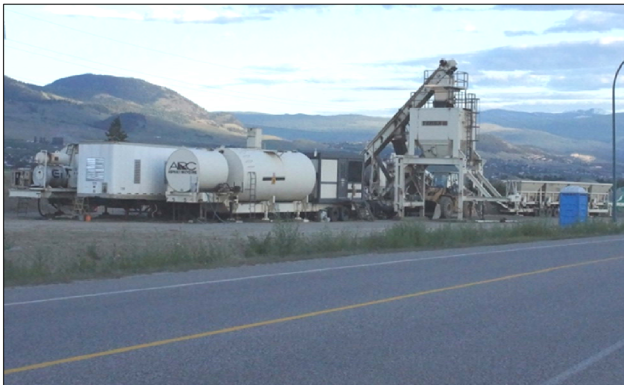
Figure 6. ARC's Terex 150 TPH, Portable Drum Mix Asphalt Plant
