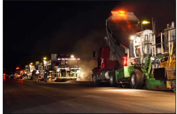
Figure 9. HIR Train From Back of Paver
