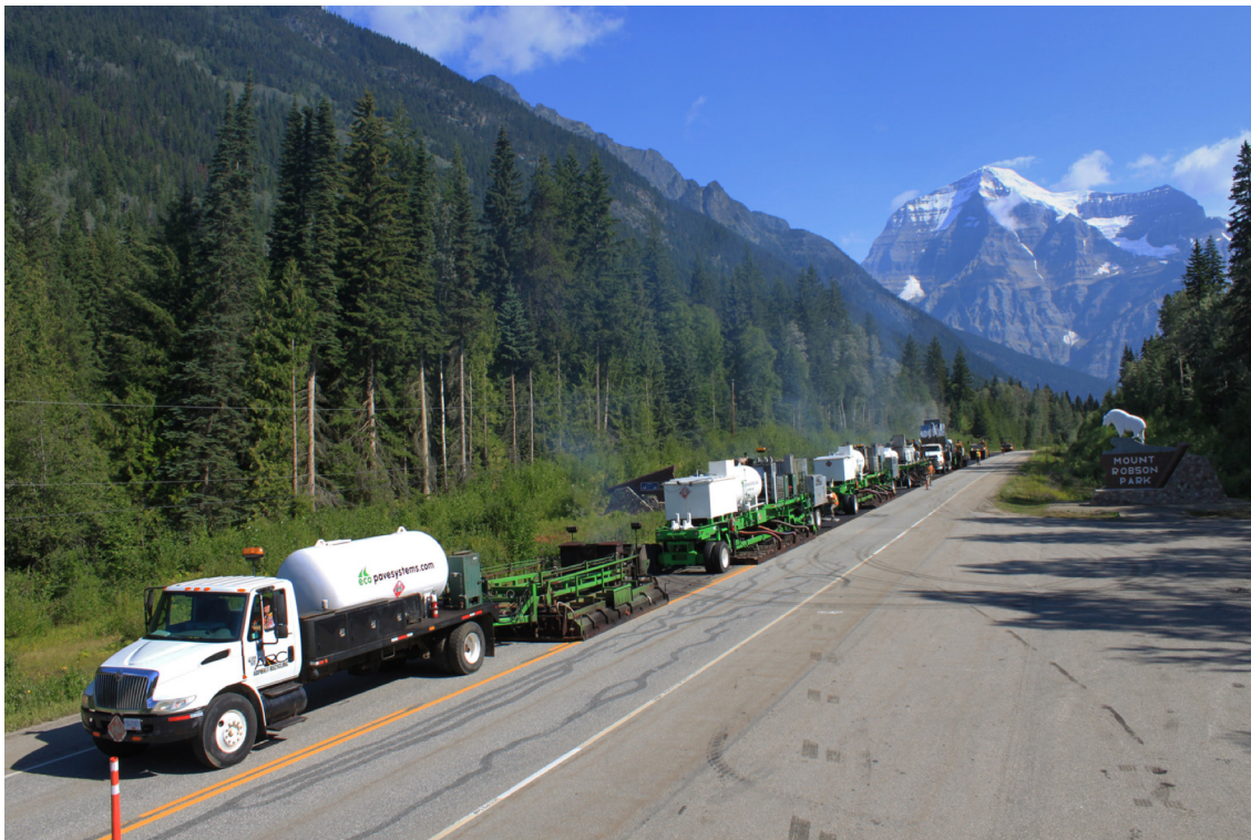
Photograph 1. Latest Hot-In-Place Recycling Train
